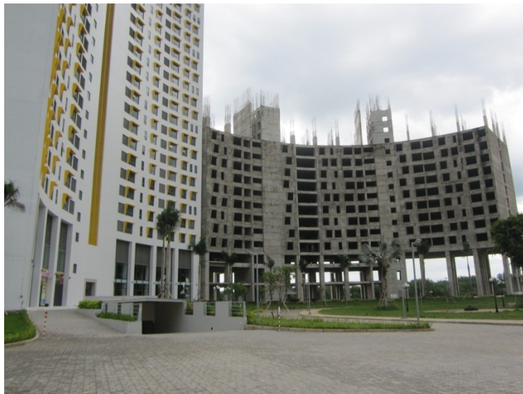
The construction of block B of The Everich 2 has hardly made progress
