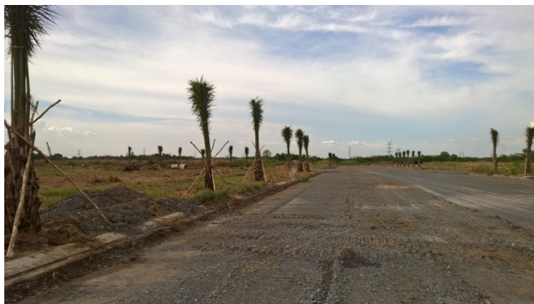
Long Thoi – Nhon Duc RA (ITC) is in the clearance and infrastructure construction process
