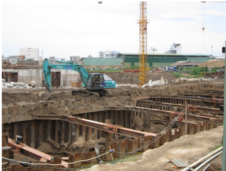
The basement of City Gate Towers will have been completed by the end of 3Q2015
