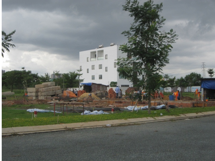
Construction of villas in Jamona City has already started
