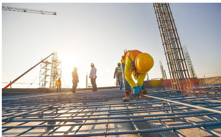
Figure 16: Steel bars for construction
