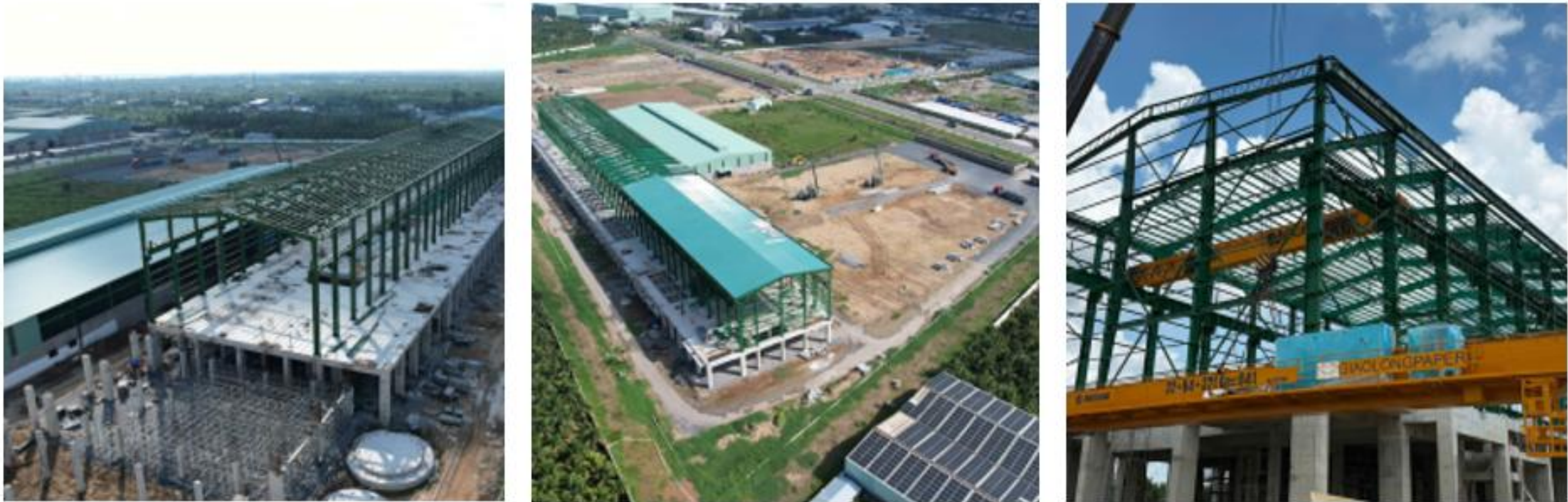
Figure 1: Progress of Key Construction and Installation Works at Giao Long 3
