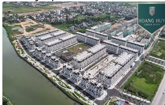
Figure 4: River Park sub-zone (HH Green River) – all low-rise units nearing completion
