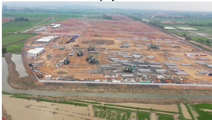
Figure 4: Que Vo 2 (Expansion) IP, with infrastructure construction for Luxshare's project cluster
