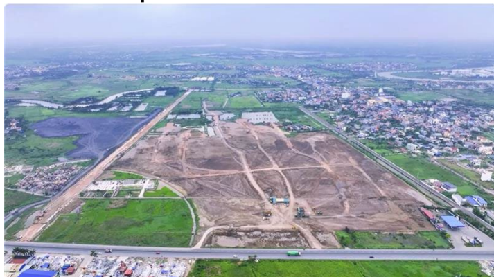
Figure 3: Trang Due 03 IP, with levelling and infrastructure construction for phase 1
