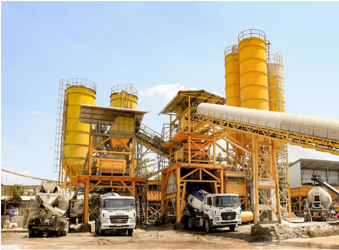
Figure 6: Concrete workshop at THG's My Tho plant
