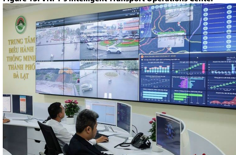
Figure 13: VNPT's Intelligent Transport Operations Center
