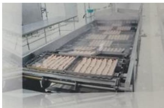
Figure 9: Steam cooking & cooling systems
