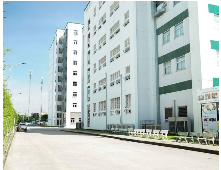
Figure 2: The high-rise RBF (phase 2) was completed in December 2025.
