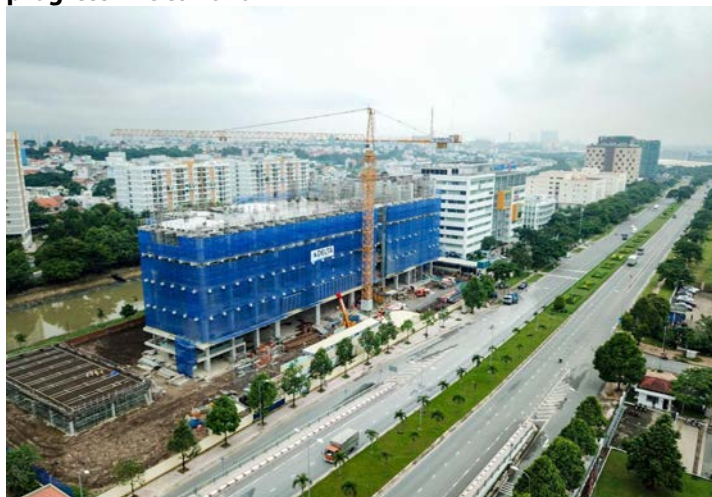
Figure 10: FOX's High-tech Park DC project construction progress in Oct-2020
